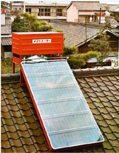
The first natural circulation system in Japan from 1963: two press-formed stainless steel sheets of 0.3 mm are seam-welded together to form a piping structure that lets water pass through it. This technology was a real exception in those days, when almost all Japanese solar water heaters were of the pipe storage type.
