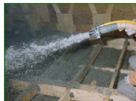
3.Blowing in the attic
